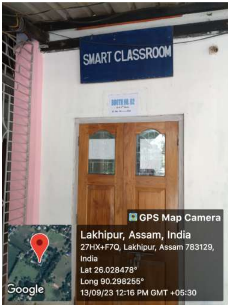
Front view of the ICT Room
